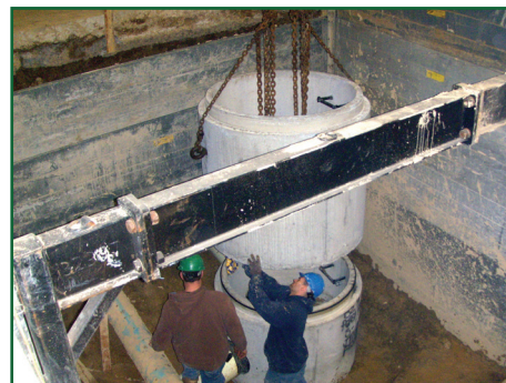
Build-A-Box with Spreader Arch
