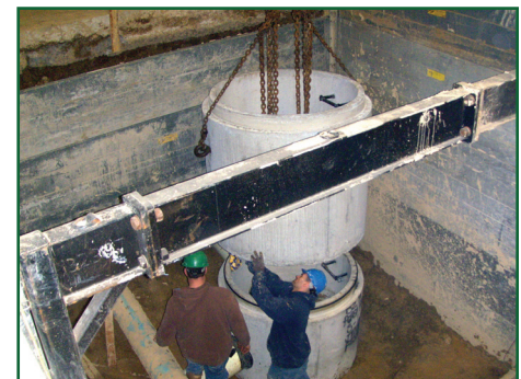
Build-A-Box with Spreader Arch
